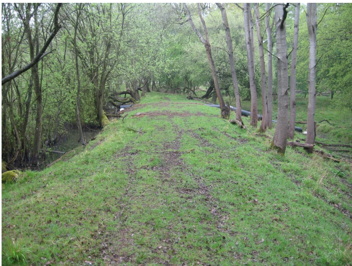
Photo 4 General view on dam, looking in a northeast direction (photo taken 08/05/2013).
